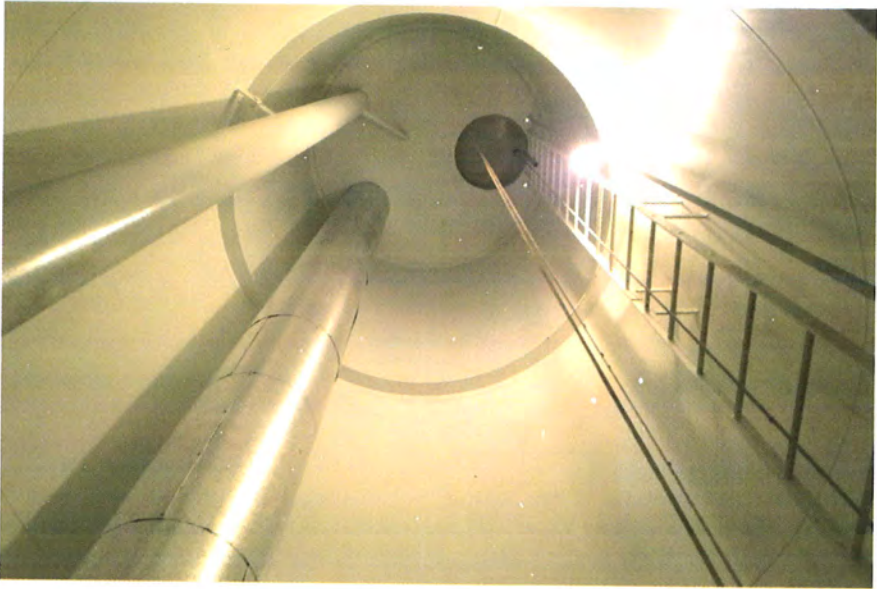
Interior dry surface is in very good condition.
